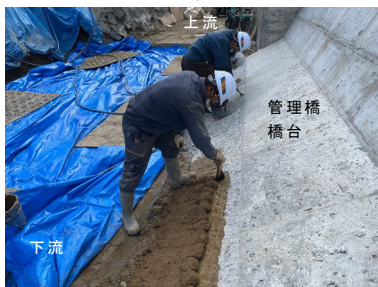
Pic.1 橋台接合部の盛立 Embankment at joint with abutment
