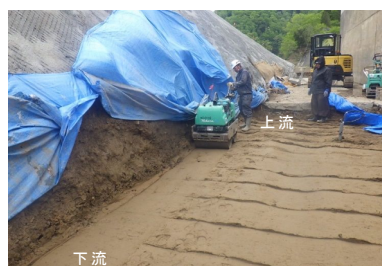
Pic.5 接合部の転圧状況(上下流) Compacting soils at joints
